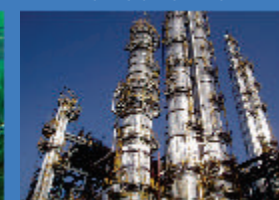
Butadiene Extraction Plant Reliance Industries Limited
